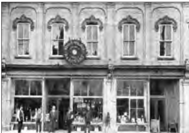
Reid & Wilson’s “Sign of the Circular Saw”.
