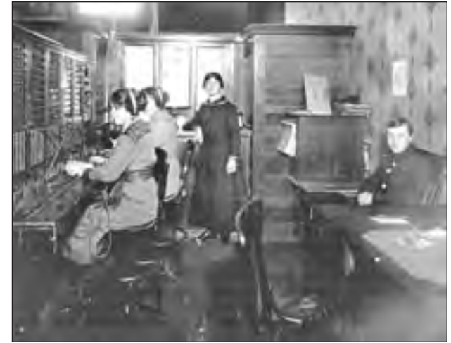
Telephone operators at the switchboard of the Bell Telephone Exchange in Seaforth's Cardno Block, 1913.
