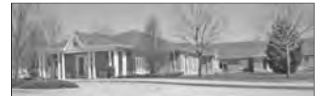
The Huronview Apartments Retirement Home.
