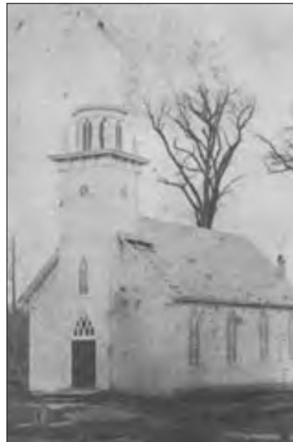
Building the Church in 1863.
