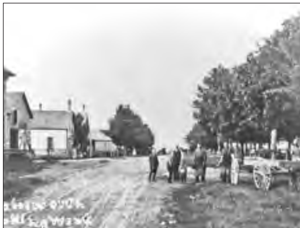
Molesworth looking west – the hotel, school (USS#4) and the general store are on the left.
