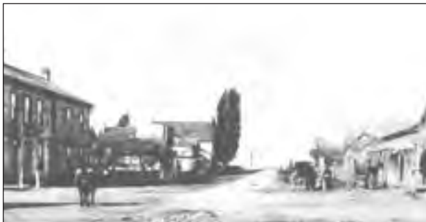
Main Street looking north: on the left are Shafer's Kippen Hotel, Mellis Blacksmith Shop, Carriage Shop, and the Methodist Church; on the right are the Post Office Store and some homes.
