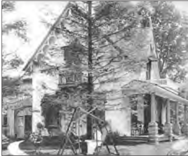
The Old Mill House is typical of the "Ontario farmhouse" style – 1½ storeys with a central gable. Note the bargeboard detail and the kingpins.
