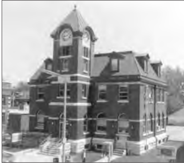
Note the rusticated stone foundation and the use of the white stone in the banding.
